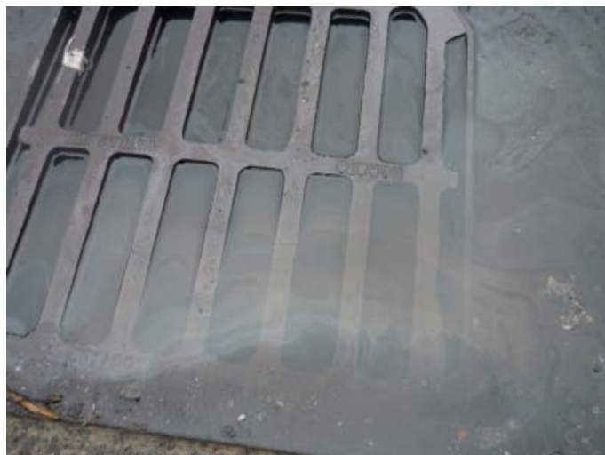
Oil sheen visible on the water surface at this blocked drain
