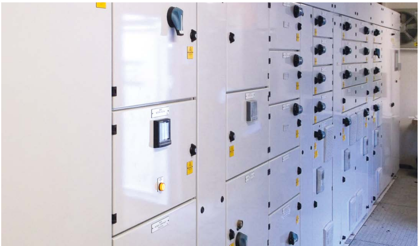
Motor Control Centre (switchboard) at a large waste water treatment works
