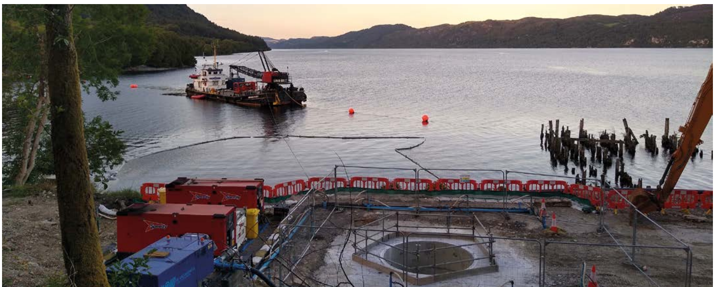
Construction of the intake pipe for Loch Ness Water Treatment Works
