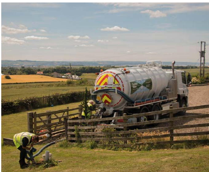
Removing sludge from a septic tank
