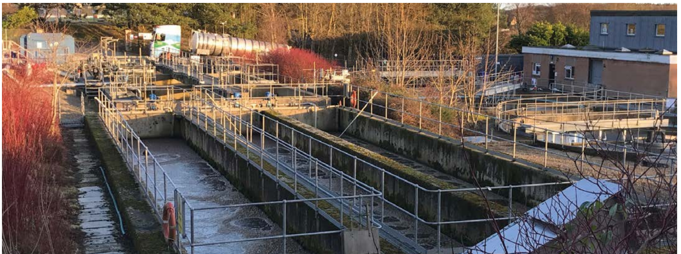
Ellon Waste Water Treatment Works showing the aeration lanes where IFAS will be deployed
