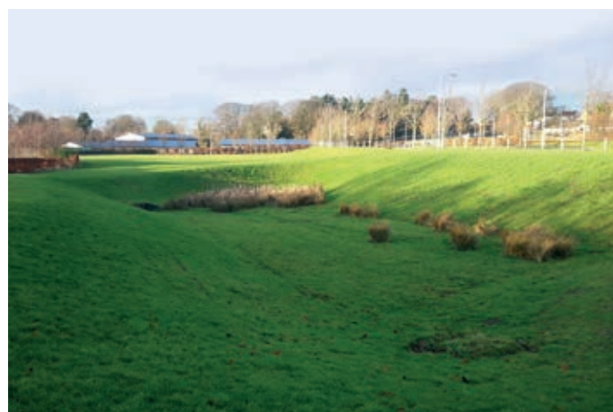
Example of a SUDS detention basin (a vegetative depression which is normally dry except during and after heavy rainfall)
