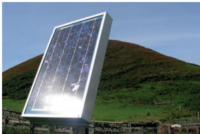
Small PV installation used to power telemetry
