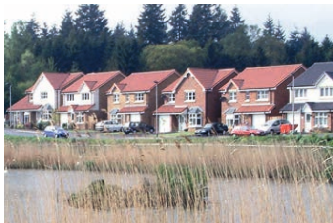
Example of a SUDS retention pond (a depression which holds water even during dry weather conditions)
