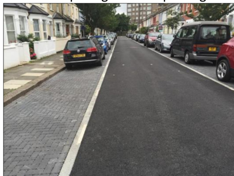
Permeable paving beneath parking
