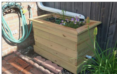
Disconnecting downpipes into planters or water butts
