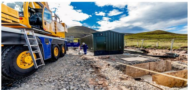
An example of a transportable water treatment unit which is currently being installed by Ross-shire Engineering in Hoy, Orkney. The proposed Water Treatment Works for Dalwhinnie will include two buildings which will be pre-fabricated and delivered to the site from Ross-shire Engineering's factory in Muir of Ord.
